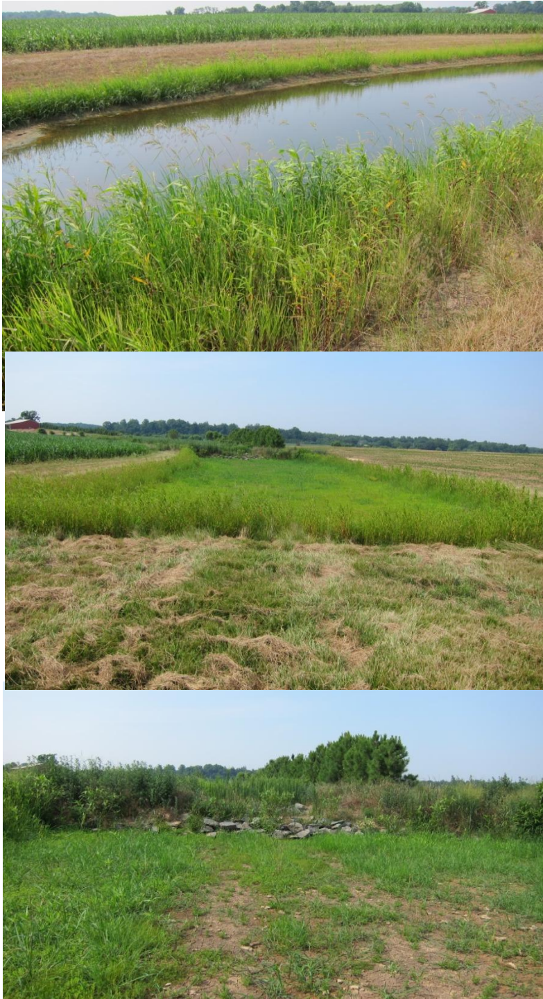
Figure 1. Photos of HIE agricultural runoff cascade treatment technology. Top: Filled basin. Middle: dry basin. Bottom: Existing outlet structure.
